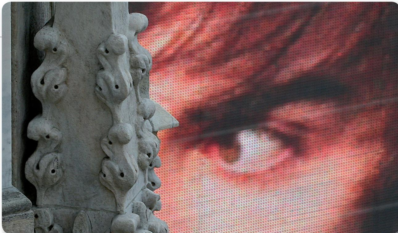
*Mediamesh<sup>®</sup>: the density of the LEDs determines the resolution of the images*
